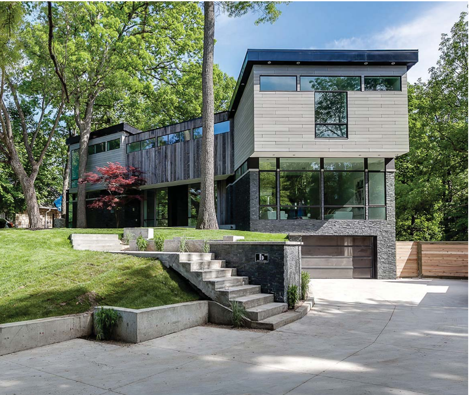
Hillside House, perched atop a hill, was inspired by the views and natural surroundings. The house feels as if it's floating within the trees.
