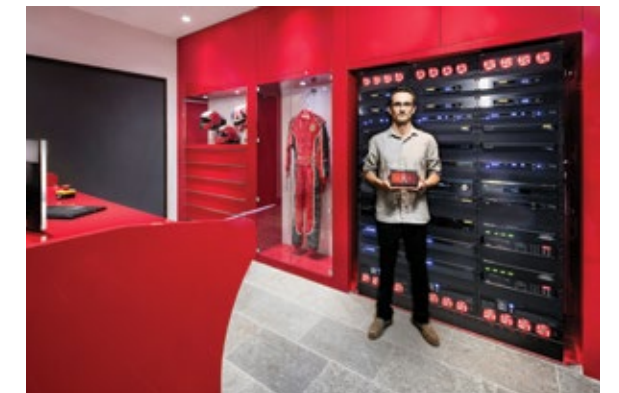
Project Installation by Lifetronic
